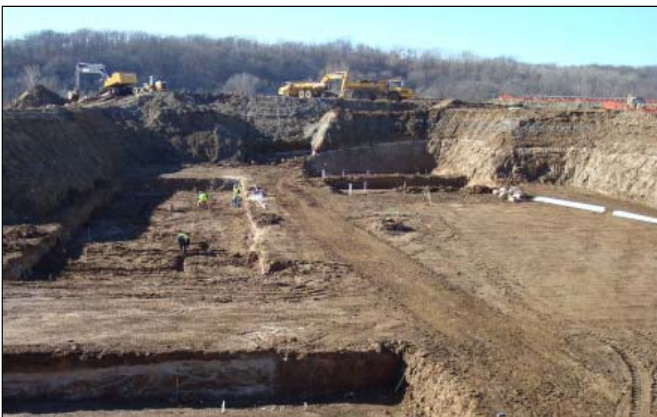
Excavated area where Operations Building will be located.
