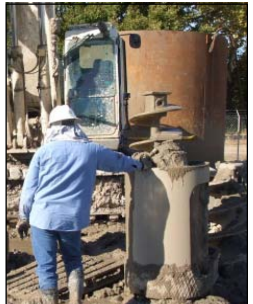
View of one of the downshafts for the Kansas River tunnel.
