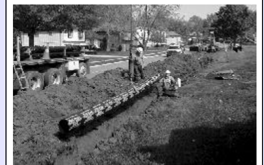
Replacement of aging water mains poses a challenge to utilities nationwide.
