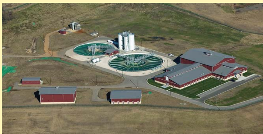
Aerial view of the Wolcott Treatment Plant
