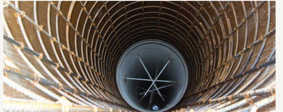
Looking down into the shaft of the Kansas River Tunnel where 60" pipe is installed.
