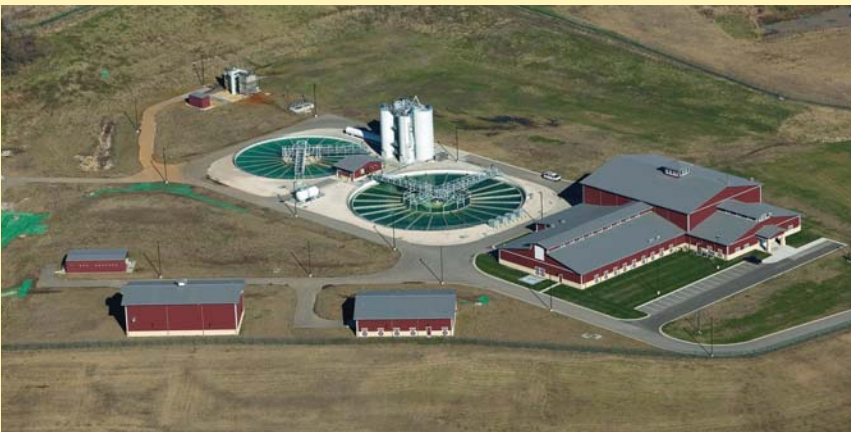
Aerial view of the Wolcott Treatment Plant
