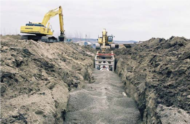
Installation of 60-inch well water supply line.
