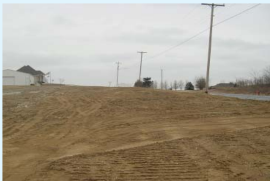
Photo showing final grading after pipe installation.
