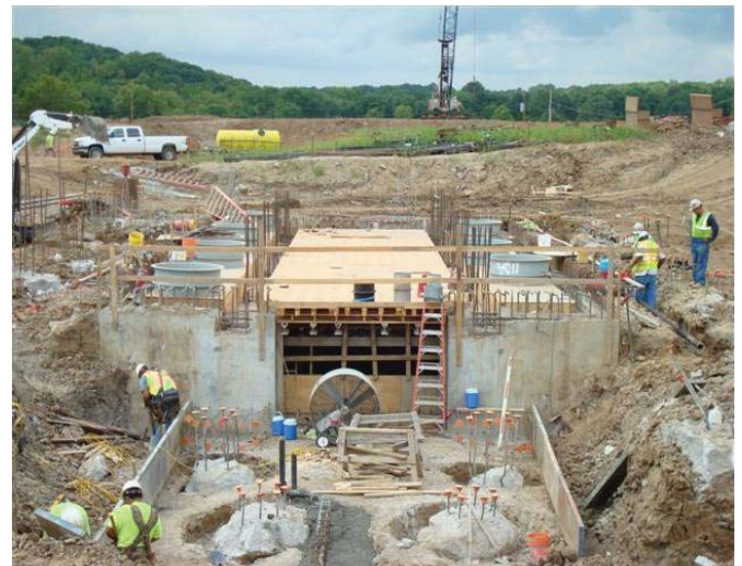
Construction of new high service pumping station.
