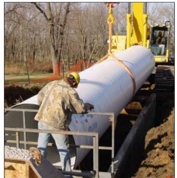
Photo showing installation of new water main.
