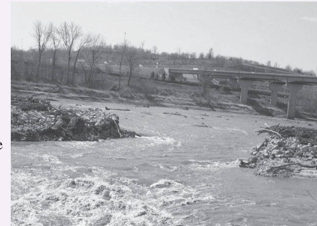
Looks west across Kansas River Jetty, showing area of break.
