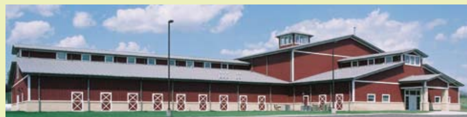
The new WaterOne Wolcott Treatment Plant
