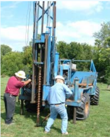
Equipment used in geotechnical drilling and survey work.
