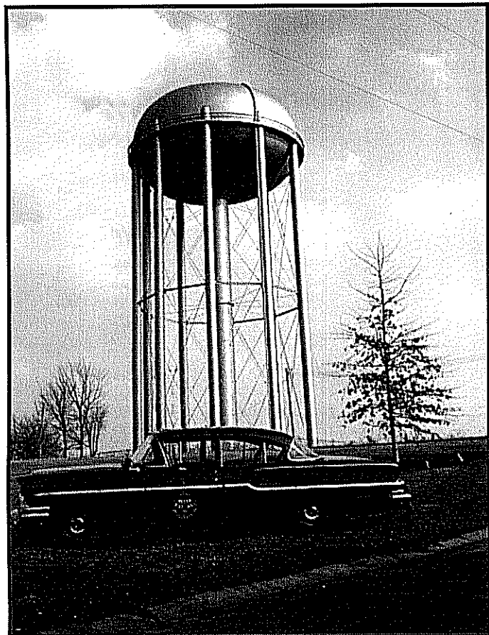
This storage tank, located at Delmar and 79 th Streets in Prairie Village, was erected in 1959; this photograph was taken in the early 1960s. Courtesy of Water One.
